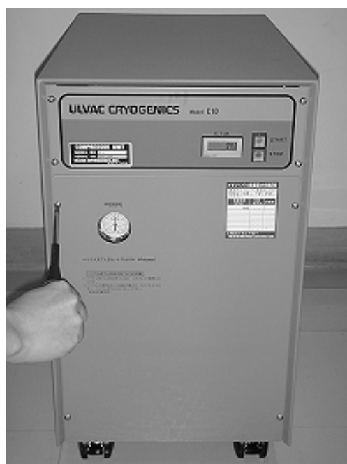
① Remove the nuts from the front panel. *Do not unscrew the screws and jam nuts on the rear panel.
