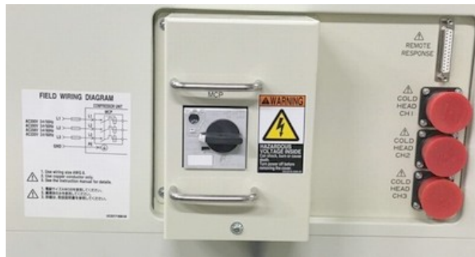
Figure 4-13 Close the Cover of Main Circuit Protector
