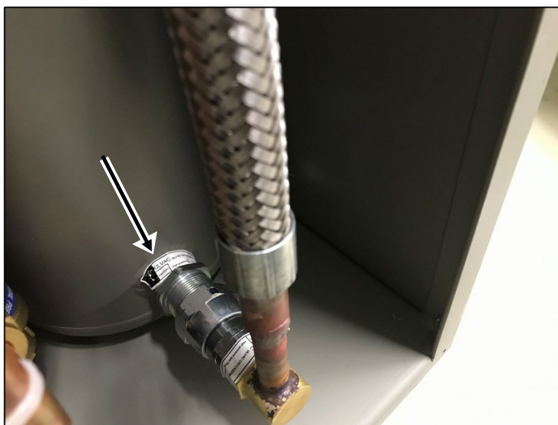
Figure Example of the sealing sticker pasted on the self-sealing coupling
