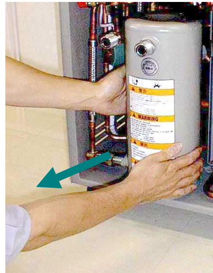
Figure 7-6 Remove adsorber mounting bolt (left)
