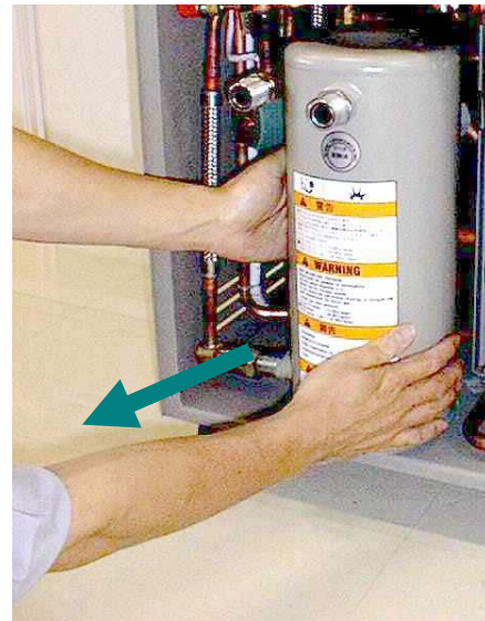
Figure 7-7 Slide adsorber outward
