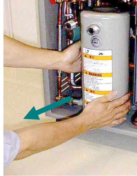
Figure 7-7 Slide adsorber outward
