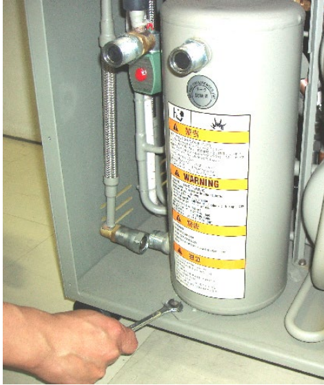
Figure 7-6 Remove adsorber mounting bolt
