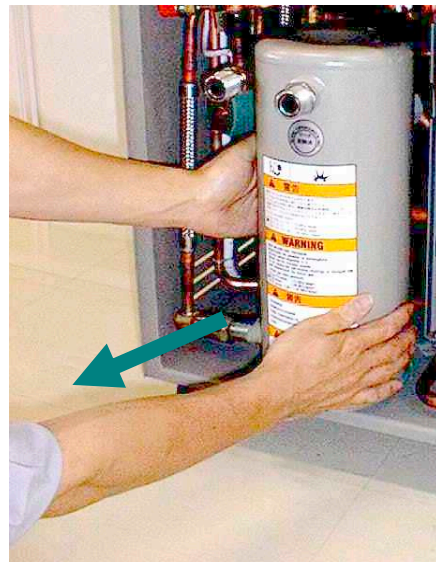
Figure 7-7 Slide adsorber outward
