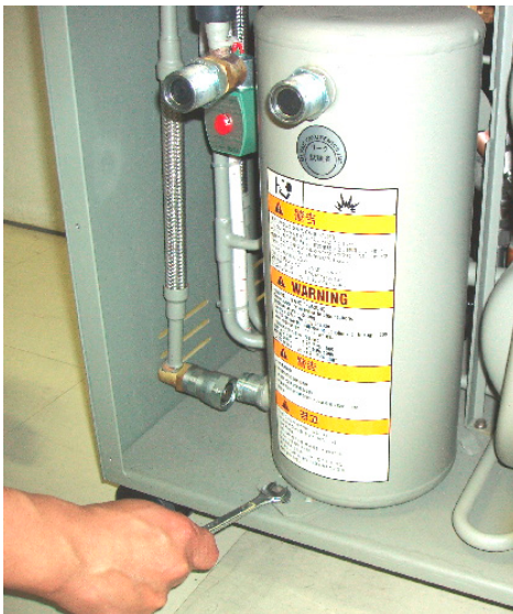
Figure 7-6 Remove adsorber mounting bolt
