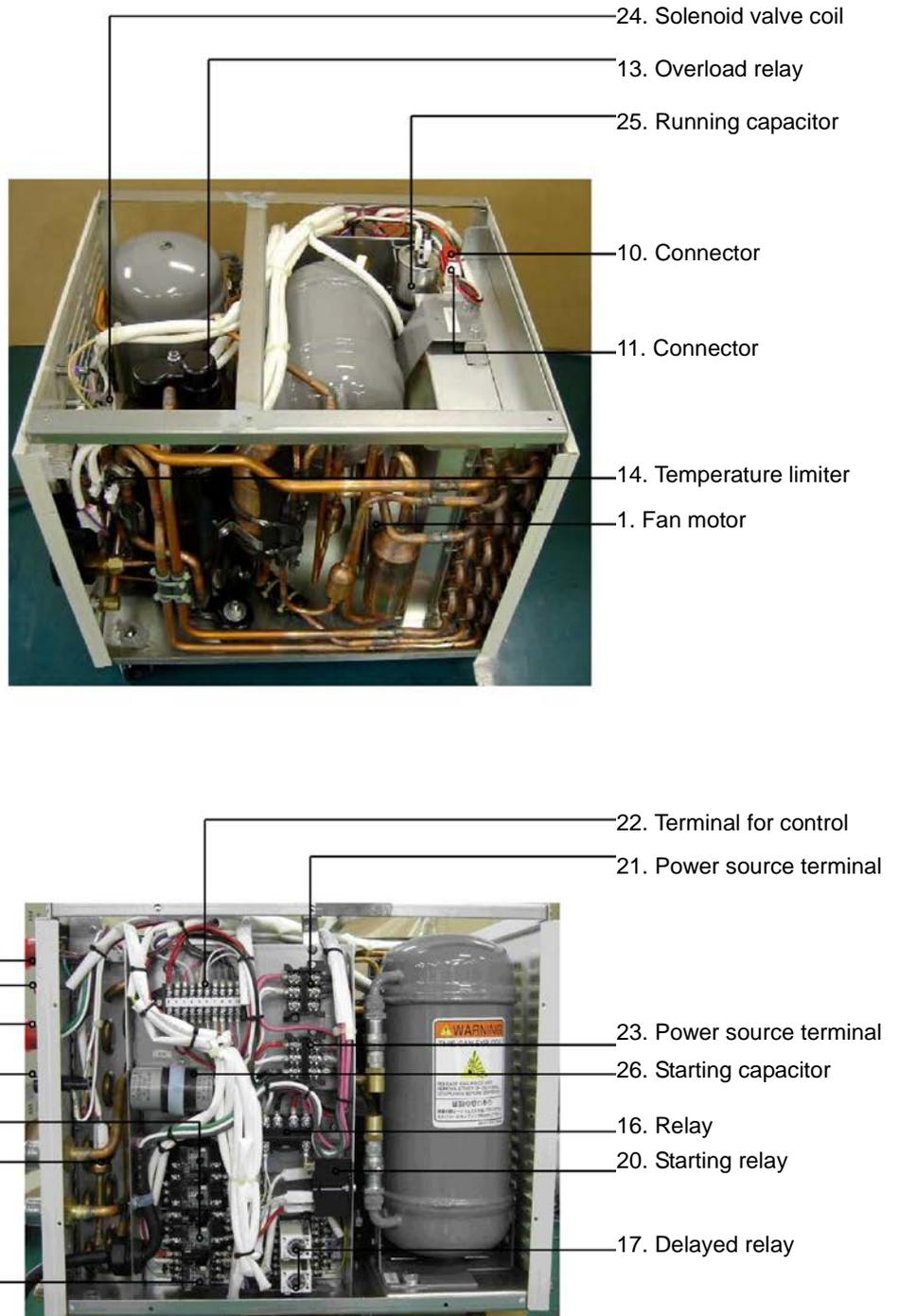
**Figure 3-5 SA112-C Control Components (interior components)**
